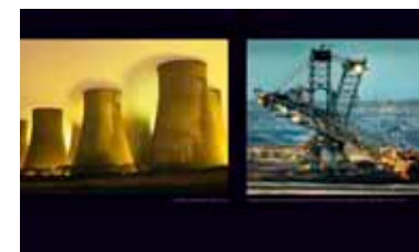
Cooling Towers: nuclear power station in Scotland; Alamy.
