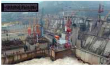
Megadam: The Xiangjiaba Hydropower Station on the Jinsha River, Sichuan province, China. China has been building large dams on its major rivers at a rate unmatched in human history; Corbis.
